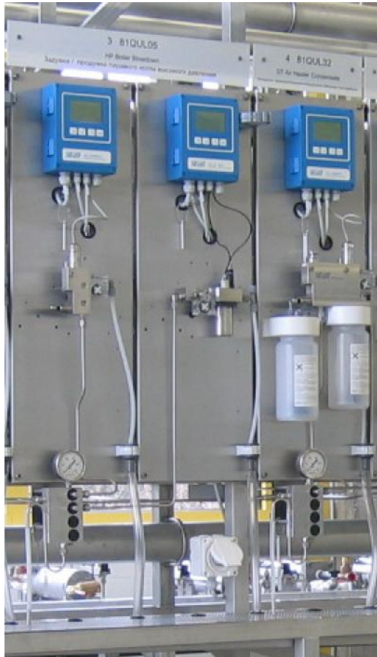
Example of SWAN Backpressure and monitor arrangement for 2 sample lines
