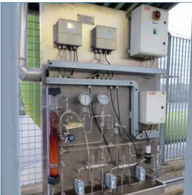
Unprotected arrangement of sensors
